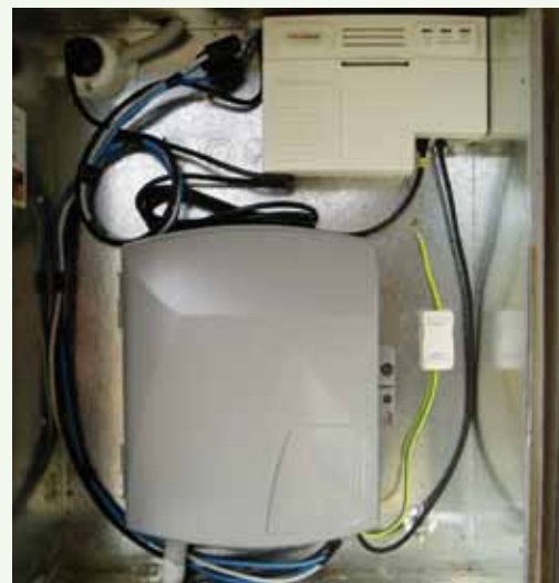
TransACT Optical Network Terminator (ONT) Installation
